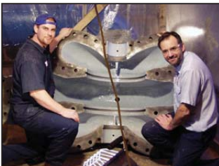
Chad Allsup and Dave Van Blarcom inspect the final coating
